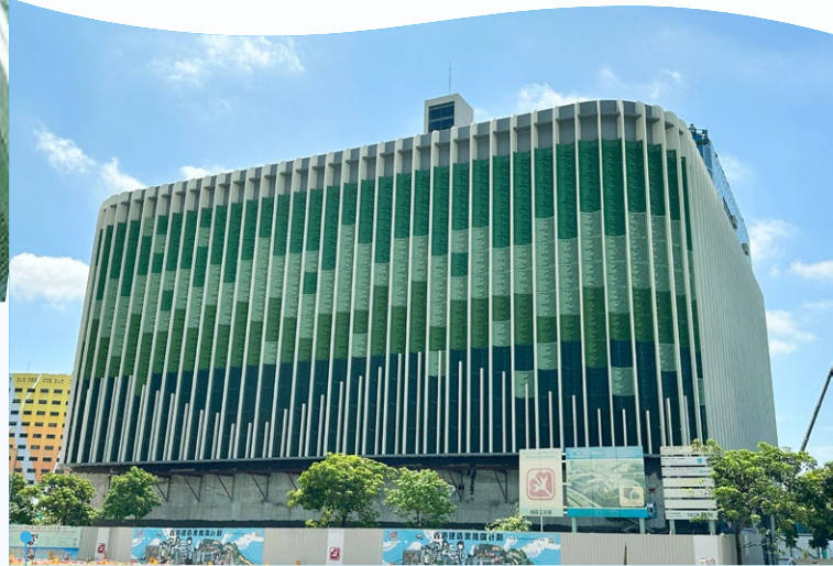
The green façade built with aluminium cladding with high recycled content. 綠色外牆由含高回收物料的鋁質面板組成。
